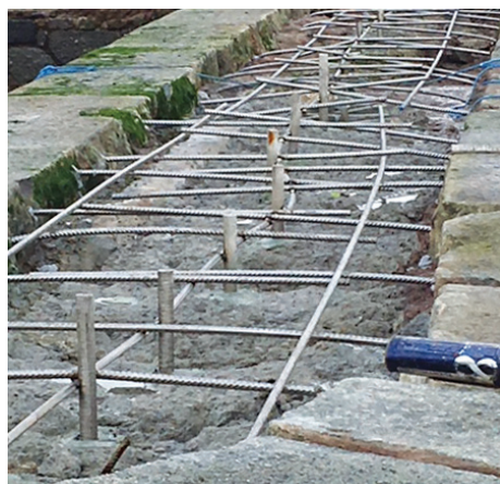
Repair method – Horizontal and vertical pinning
