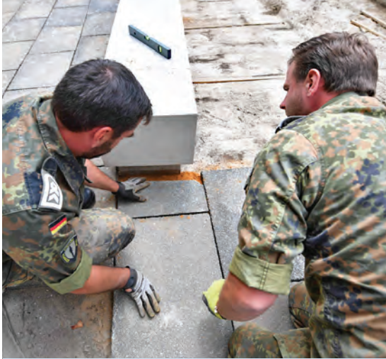
New paving slabs were painstakingly prepared and positioned.
