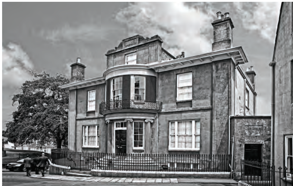
Bonamy House - designed and built for John Collings in 1817. (photo: Graham Jackson, © Blue Ormer)
