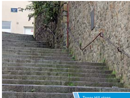
Tower Hill steps.
