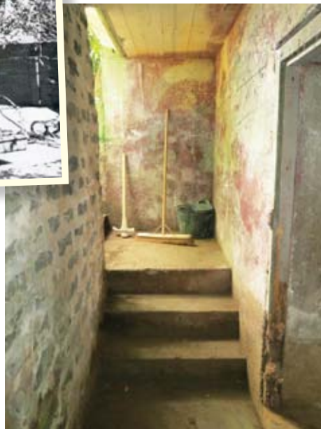
Ammunition bunker before and after excavation. Note the original camouflage paint.
