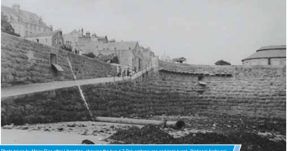
Photo taken by Major Rice after Liberation, showing the two 4.7 Pak embrasures and tank turret. (National Archives)
