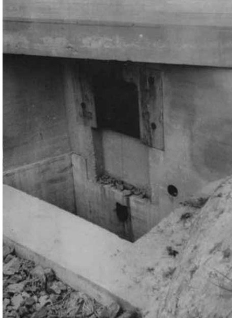
Photo taken by Major Rice after Liberation of a type 676 bunker for 4.7 Pak viewed from the front showing the spent shell pit and armoured shield in the raised position. (National Archives)
